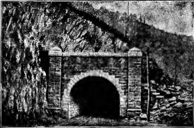
FIG. 49. — East Portal of Hoosac Tunnel.
